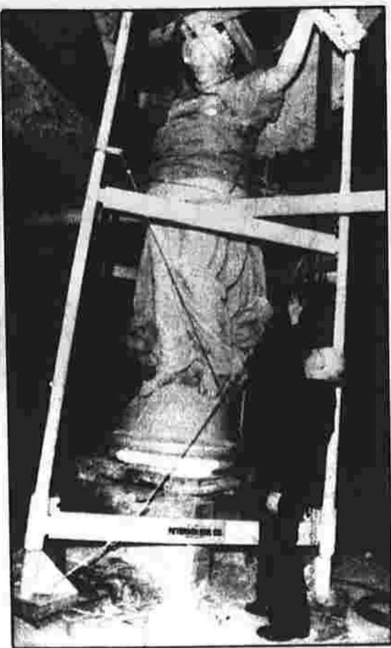
The Rev. Joseph A. Davine, chairman of the state Commission on Capitol Preservation and Restoration, stands next to the "Genius of Connecticut," damaged during restoration work.
